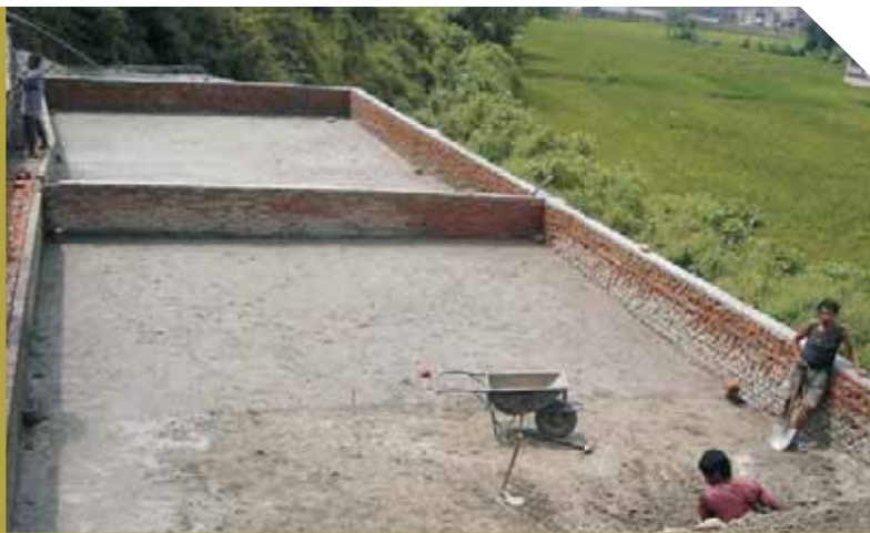
Basin ready for lining and filling of substrate
