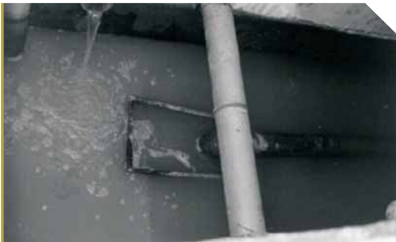
Feeding tank and mechanism - Bucket sinks down and water flushes into the bed (Shrestha R.R., 1999)
