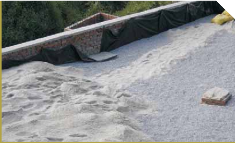
Filling of substrate (main layer) in vertical flow CW
