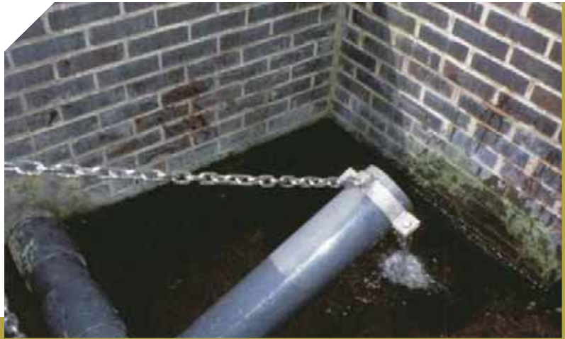
Swivelling elbow outlet (Cooper et al. , 1996)
