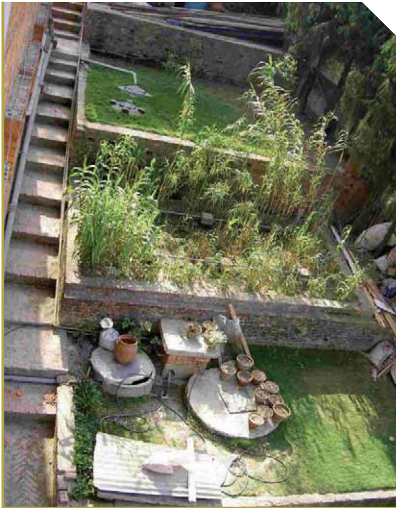
Constructed wetland at ENPHO
