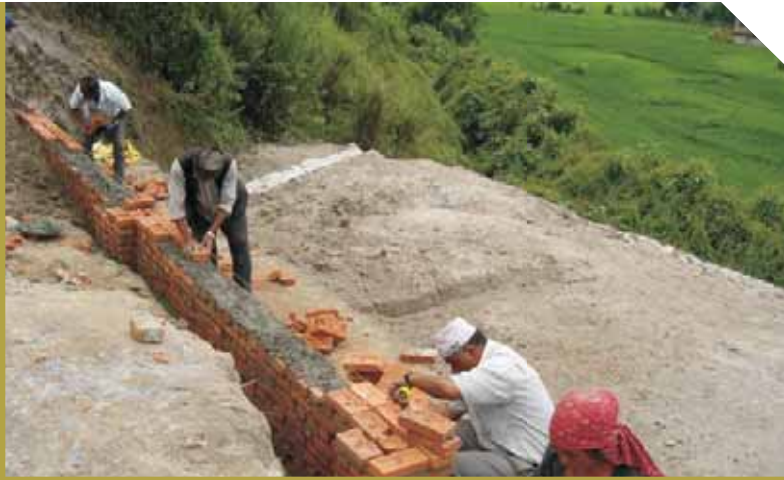
Construction of walls of the basin
