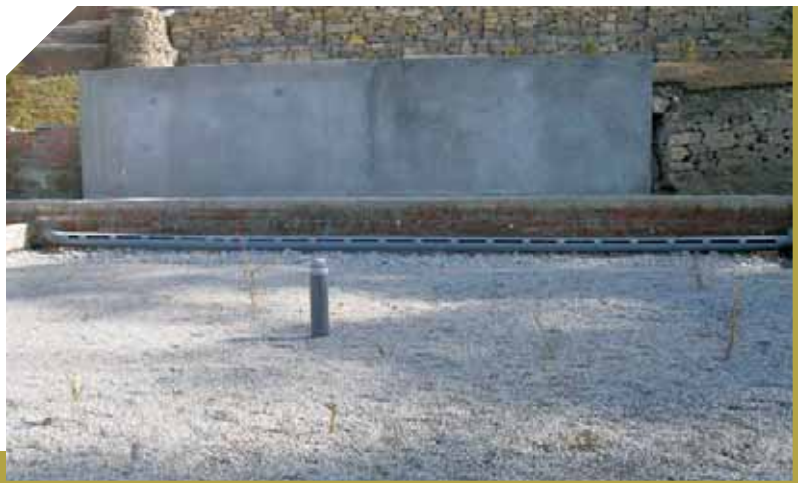
Horizontal flow CW after completion and plantation of vegetation
