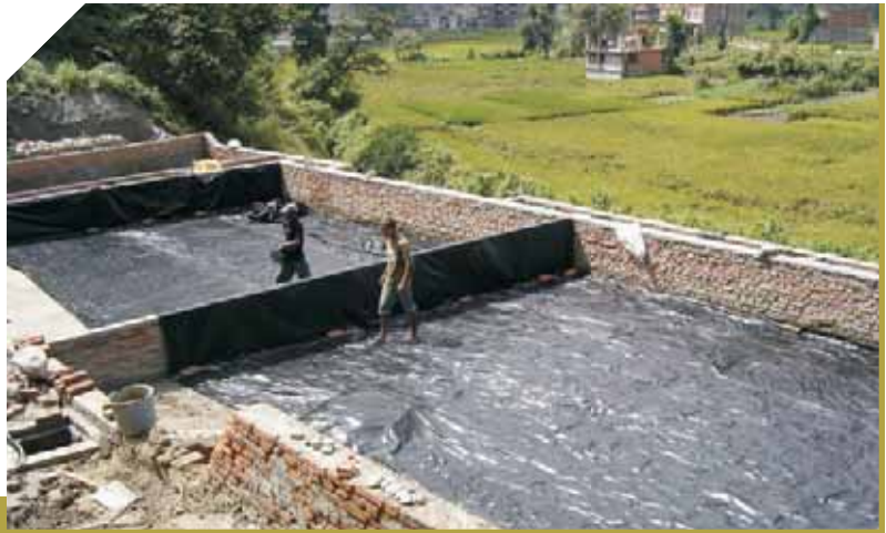
Plastic liners placed in the basin
